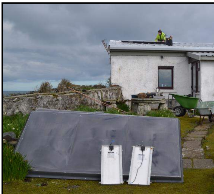
Old solar hot water & PV panels removed from roof
