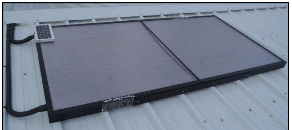
Solar hot water and PV panel installed on roof
