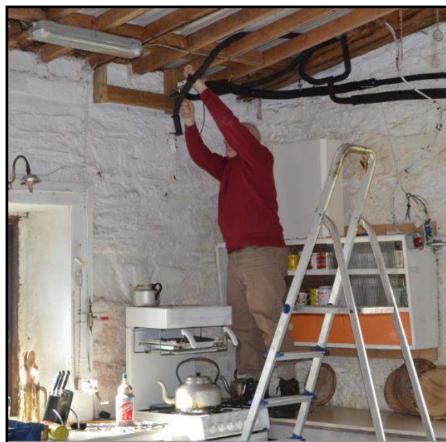
Larry dismantling old hot water system
