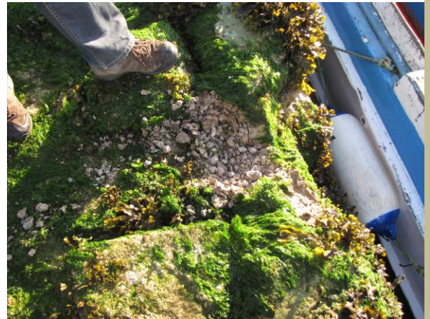
Crumbling concrete on the South Jetty
