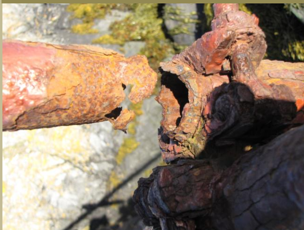
Some of the rotten steelwork on the East Jetty – see page 3
